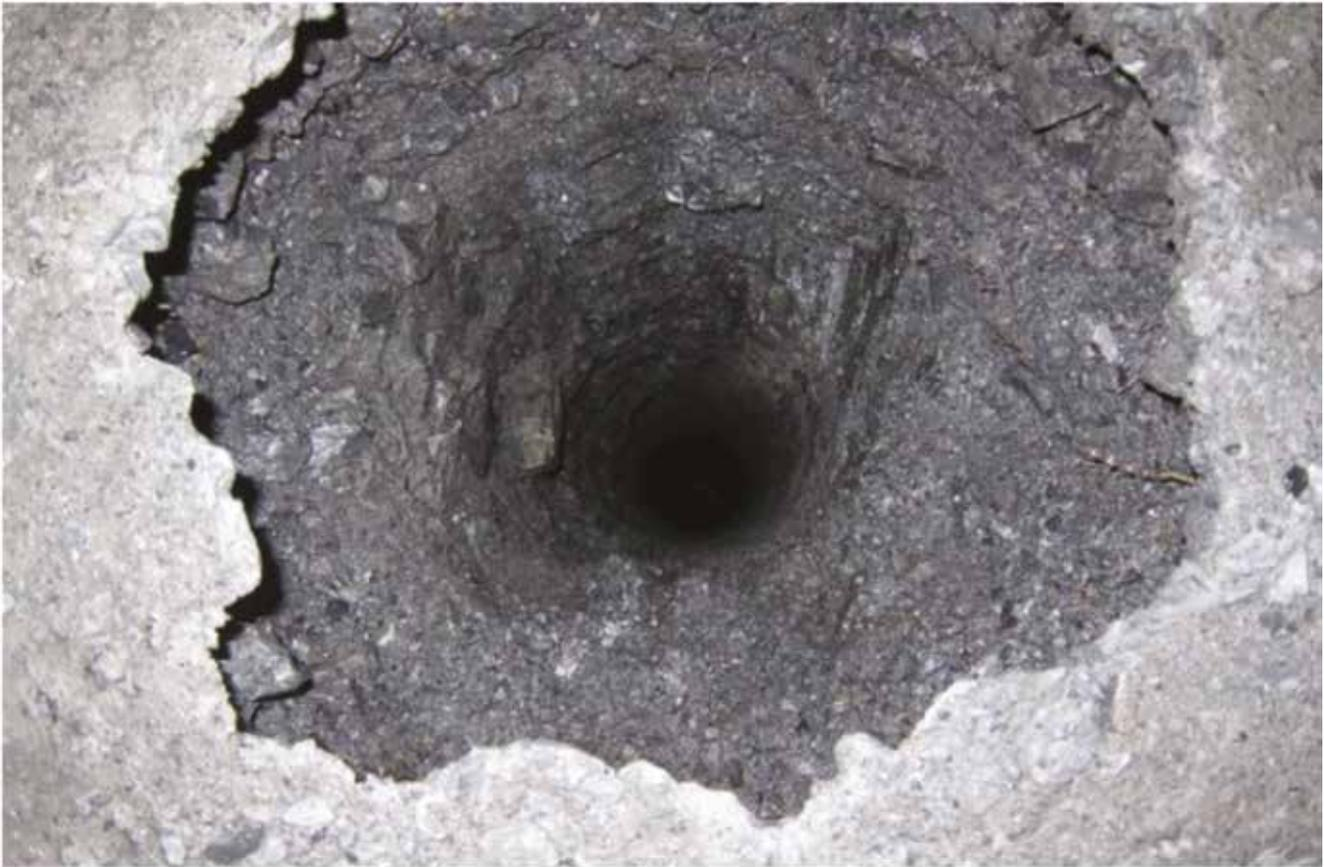
Figure 2. Slot raise drilled by Rhino 100.
